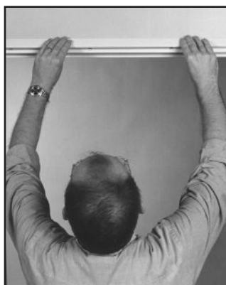
7 Snap on header casing.
