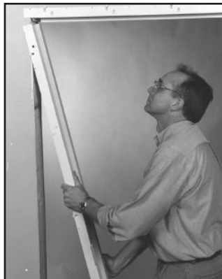
3 Set strike jamb over wall section.
