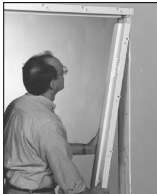
2 Set hinge jamb over wall section.
