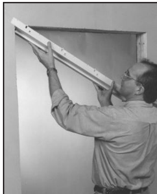
1 Set header over wall section.
