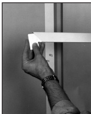
6 Slide corner backing angles into header casing.
