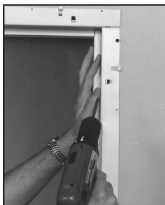
5 Apply fasteners starting at upper end of hinge jamb.
