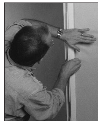
8 Slide jamb casing over corner backing angles. Align with jamb clips then snap on casing.
